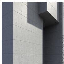
Wall of exposed concrete; 2x2 panel shuttering
