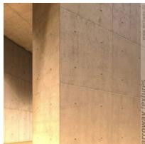
wall of exposed concrete; 2x2 panel shuttering; corresponding to 'concrete 23' and 'concrete 25'
