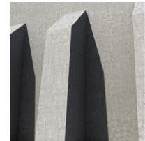
Concrete wall with block structure created by the shuttering
