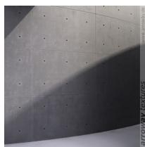
wall of anthracite colored exposed concrete; 3x2 panel shuttering; corresponding to 'concrete 26' and 'concrete 27'
