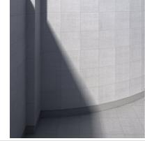
Concrete slabs with textile-like surface
