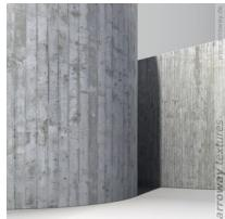
wall of exposed concrete; distinct boards-structure, created by the shuttering
